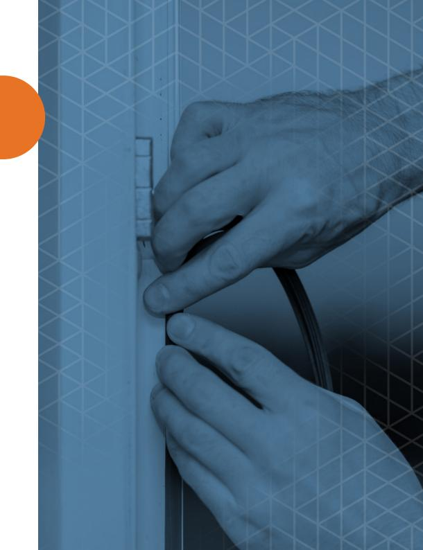
There are several options for homeowners to replace that insulation. If it's a big gap, they can cut strips of fiberglass insulation or backer rod (a cylindrical type of foam) and insert them into the opening. They must make sure not to force the materials into the space because that could bend the window or door frame.
